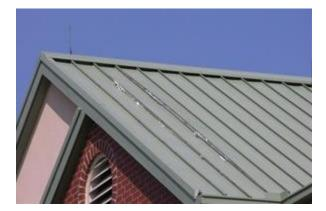
To install this LPS on a ridge, the conductor was placed under the ridge cap, shielding it from the wind. Flashing was required where the air terminal penetrates the cap. (Photo courtesy of TL Smith Consulting Inc.)
